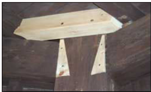
The reconstruction has been left uncolored in order to discern original craftsmanship from the repairs.
